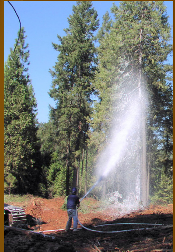
Outside Hose Lay
